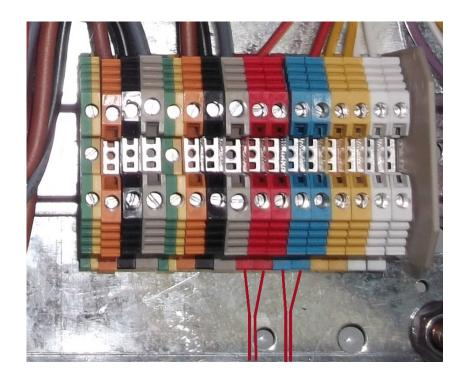
If only a single device is used then ignore the centre 2 terminals and connect across the outer 2 terminals as shown below.
